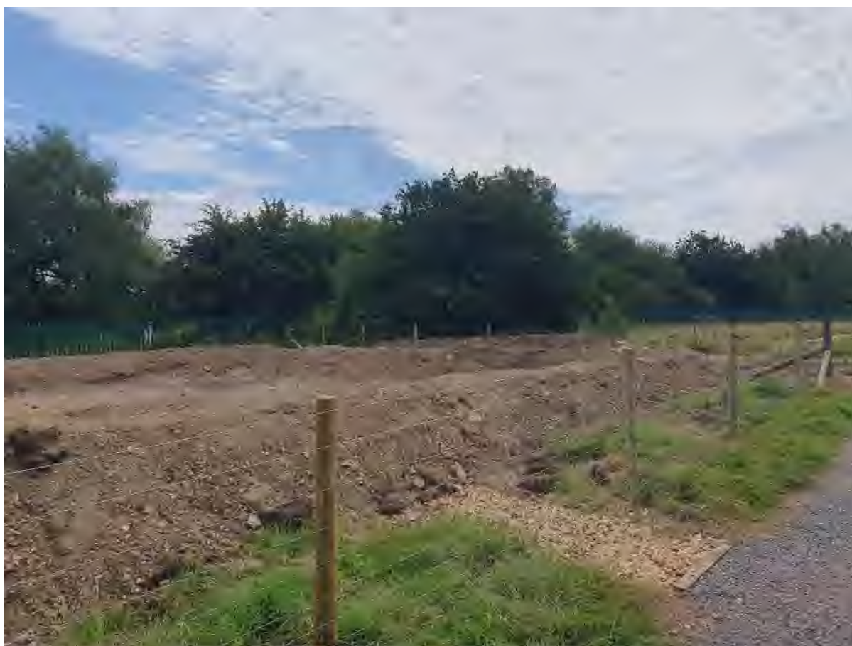
Figure 1 - Photo of new retention pond
