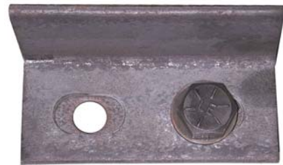
Fig. 2 View showing oval holes over round holes with one of the keeper bolts removed.
