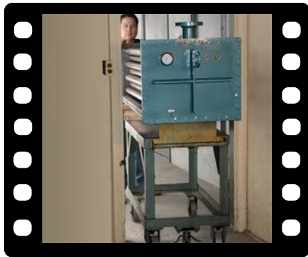
Largest Piece: 50 Horsepower Boiler Pressure Vessel going through 34" wide door (From RITE Take-A-Part Video)
