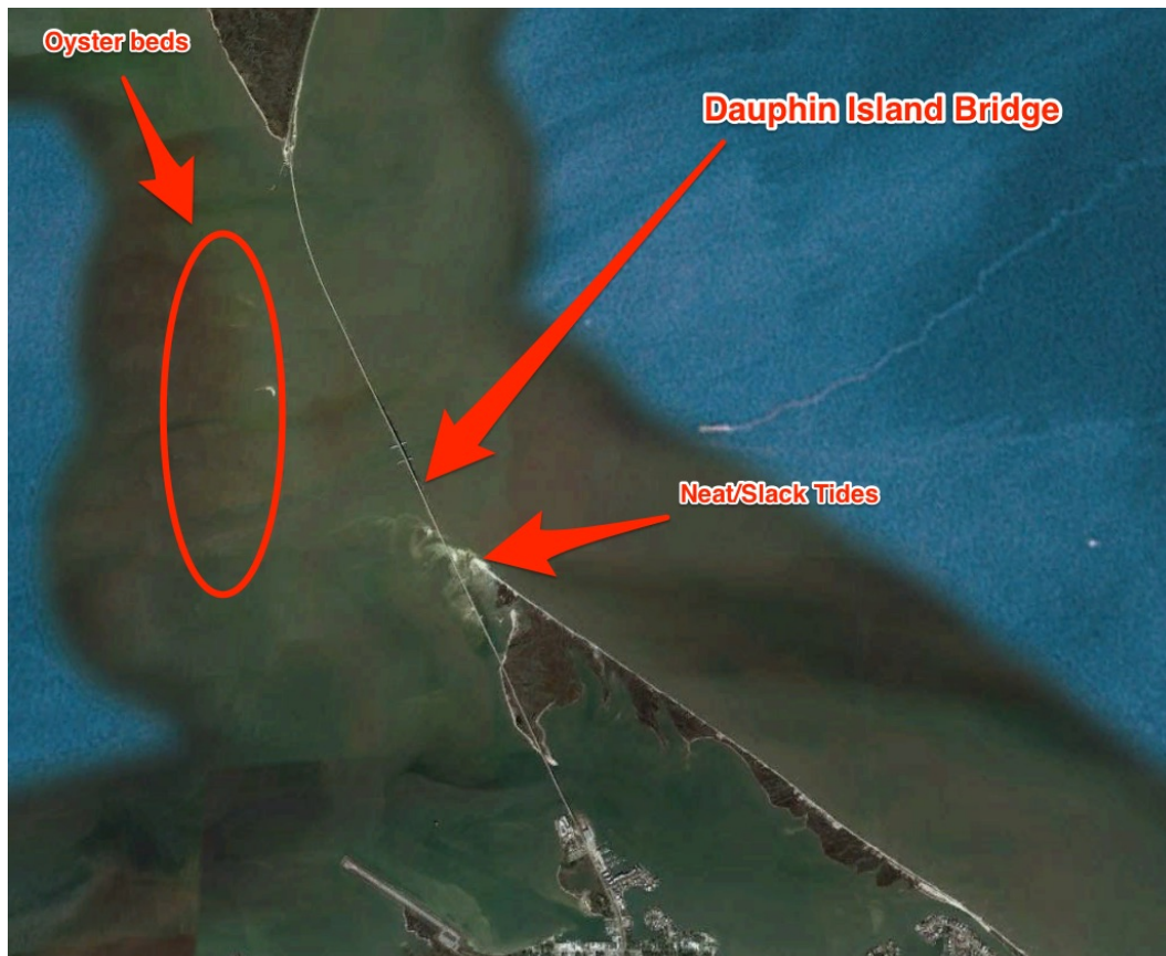
FIG 3.1 - DAUPHIN ISLAND BRIDGE
