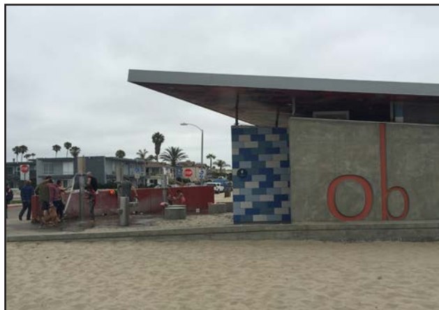
Ocean Beach public restrooms and showers.
