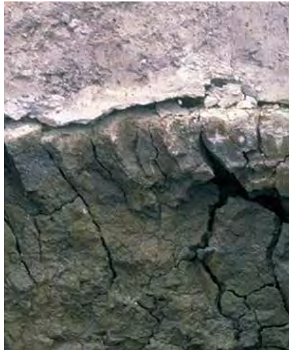
Figure 6.16. A sodic soil in Tasmania, Australia, that lacks aggregation and has problems with waterlogging when wet and with hardsetting when dry. Photo by Richard Doyle.
