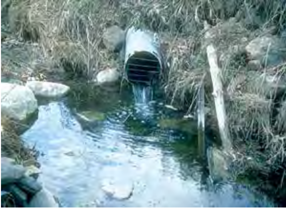
Figure 17.20. A subsurface drain line discharges into an edge-of-field ditch, diverting groundwater to surface waters.
