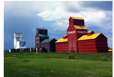
R-PS80-1272-254, Grain elevators in Grayson, SK, 1980
