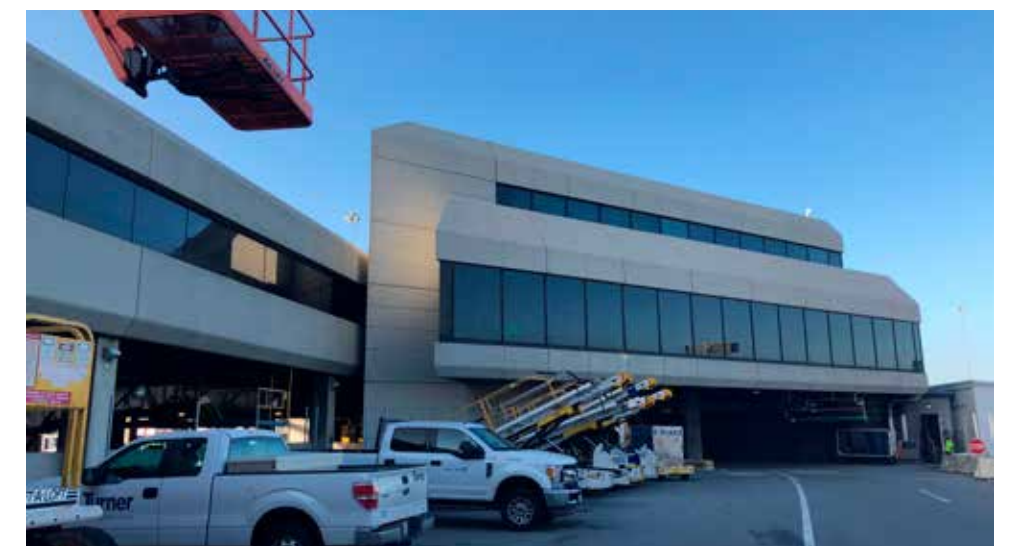
C. EXISTING FACADE
