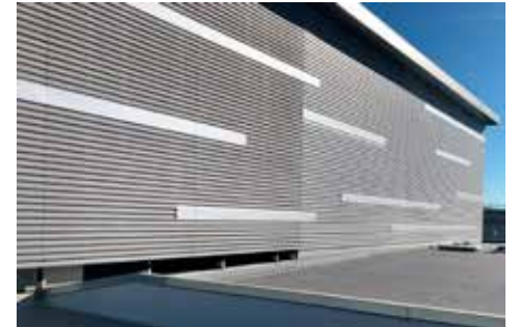
CORRUGATED / PERFORATED METAL PENTHOUSE (TERMINAL 3 EAST)
