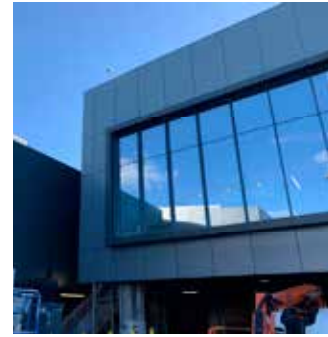
METAL BROW SURROUND (TERMINAL 3 EAST)
