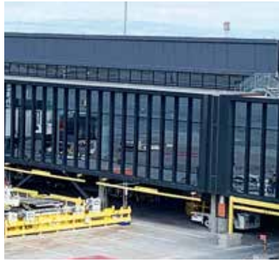
DARK METAL PANEL (T3 BOARDING AREA E)
