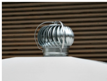
A wind-driven roof turbine
