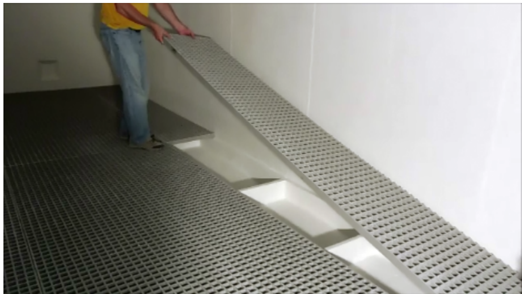
Sectioned area of containment floor to sit below shower area
