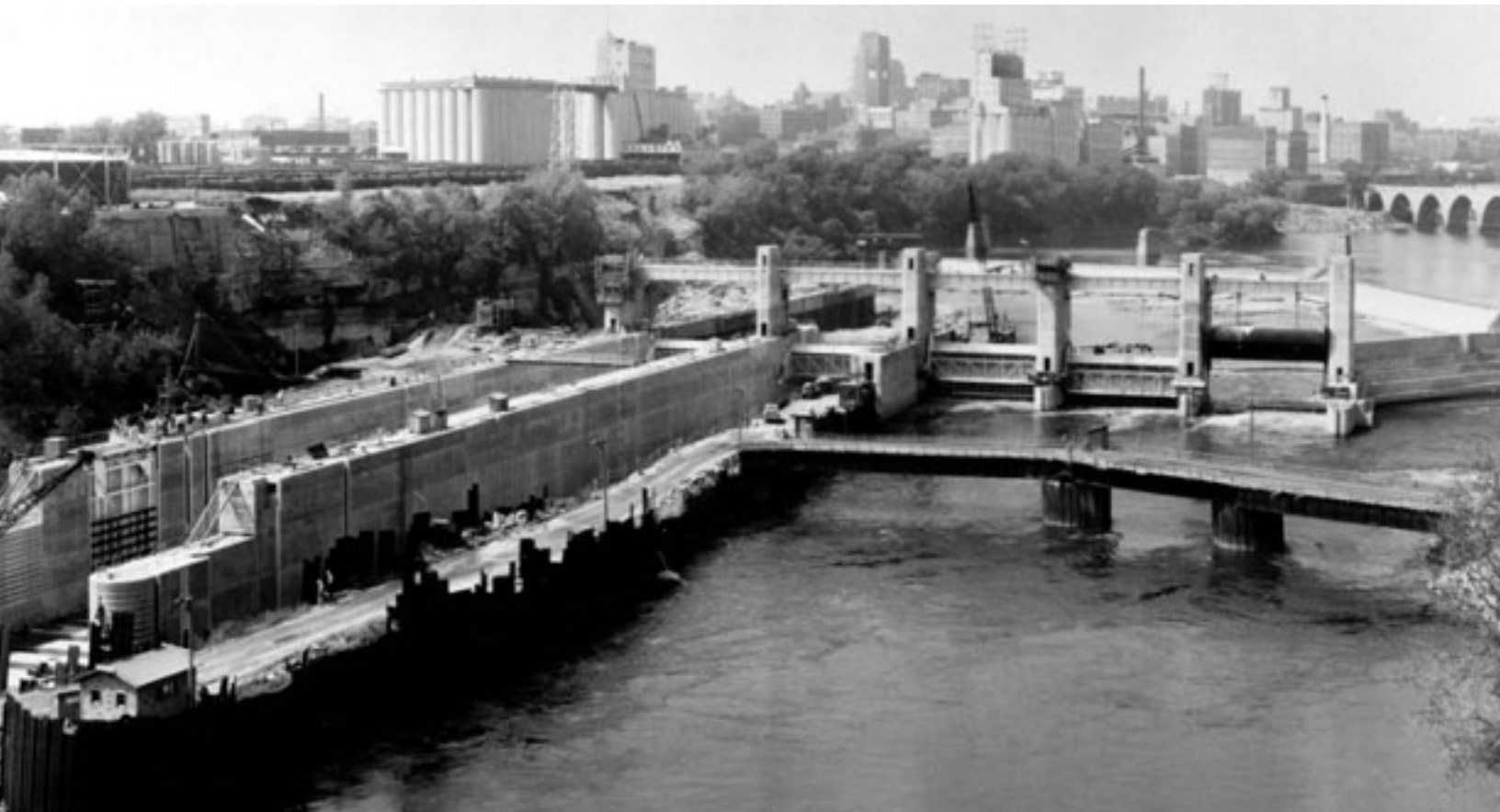
FIGURE 9. Lower St. Anthony Falls Lock and Dam under construction, 1956. St. Paul District, Corps of Engineers.
