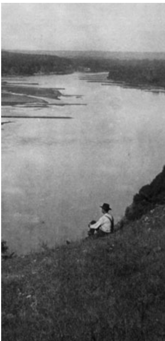
FIGURE 2. Detail, Wingdams below Nininger, Minn., 1891 . By Henry P. Bosse. St. Paul District, Corps of Engineers .
