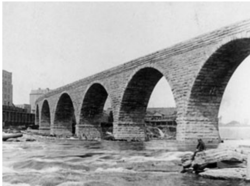
FIGURE 10. James J. Hill's Great Northern, Stone Arch Bridge, 1884.
