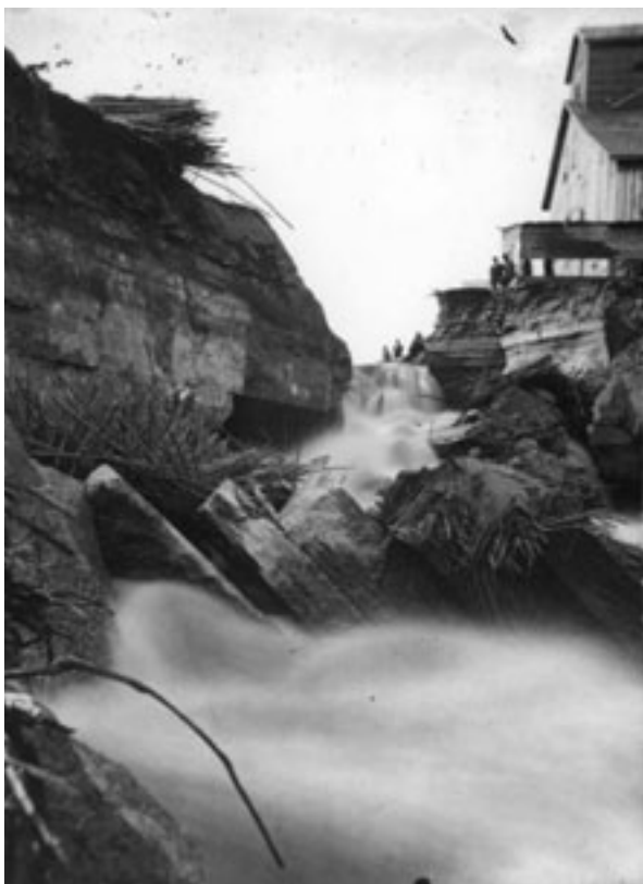
FIGURE 7. Eastman Tunnel collapse, Hennepin Island, 1869. Minnesota Historical Society.
