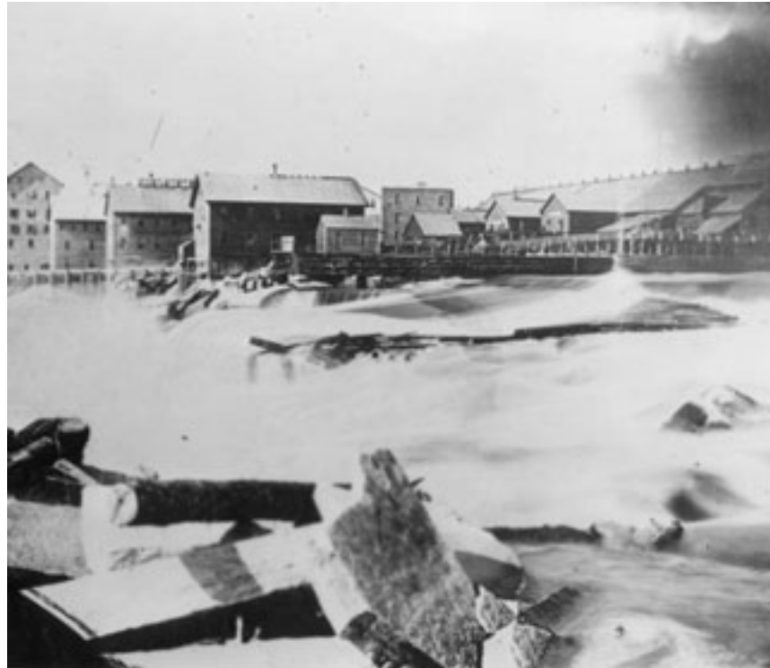
FIGURE 6. West side platform mills, about 1868. Photo by Jacoby. Minnesota Historical Society.
