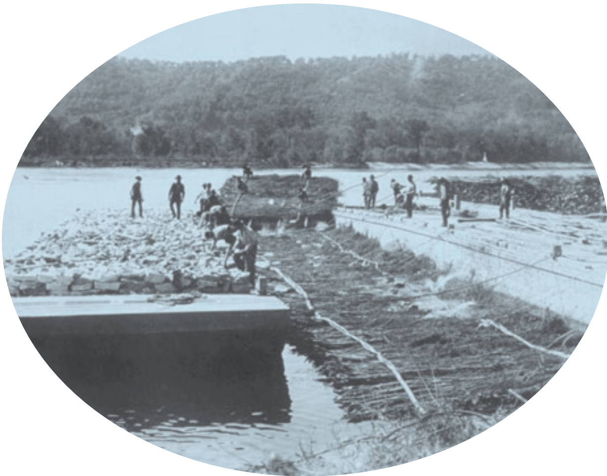
FIGURE 9. Wing dam construction. Photo by Henry P. Bosse. St. Paul District, Corps of Engineers.
