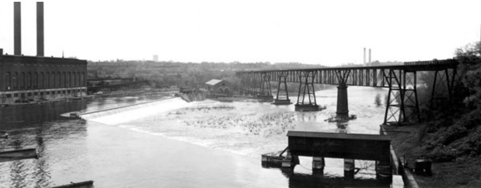
FIGURE 6. De la Barre's "folly." Lower St. Anthony Falls Dam and Hydroelectric Station, completed in 1897. St. Paul District, Corps of Engineers. The Twin City Rapid Transit Company steam powerhouse is at the far left. University of Minnesota Steamplant is at the far left.
