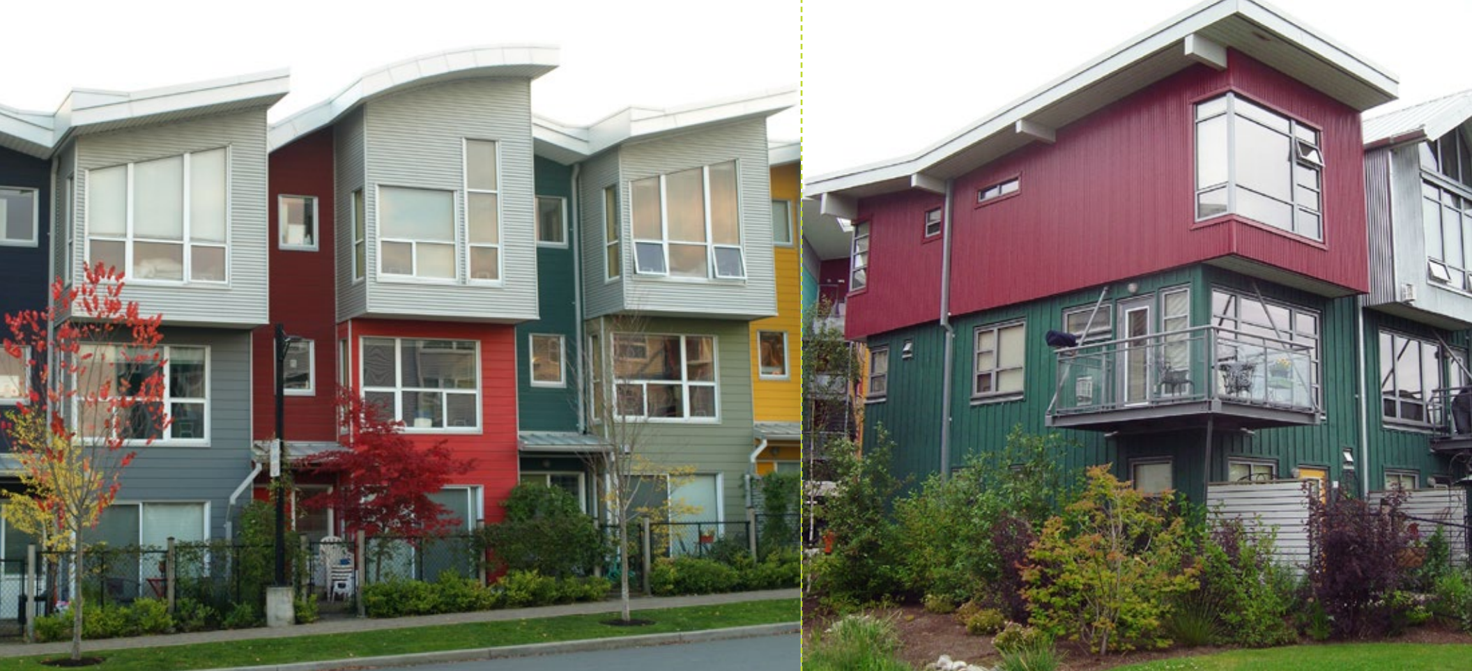
Figure 14: Example of buildings using diverse materials
