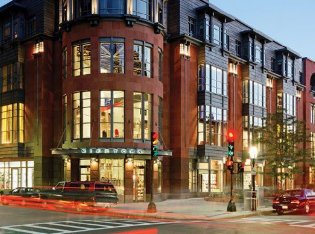
Figure 17: Example of building with corner entrance
