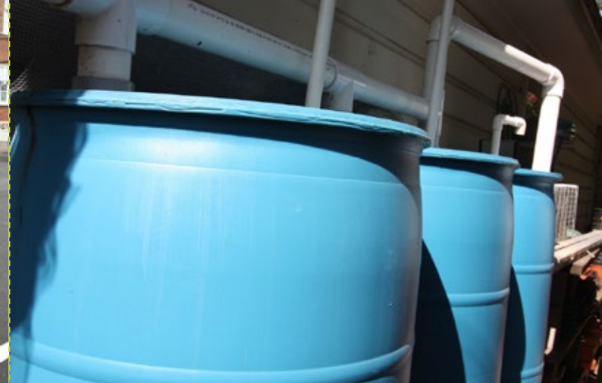
Figure 22: Rain barrels are an easy way to allow the reuse of water
