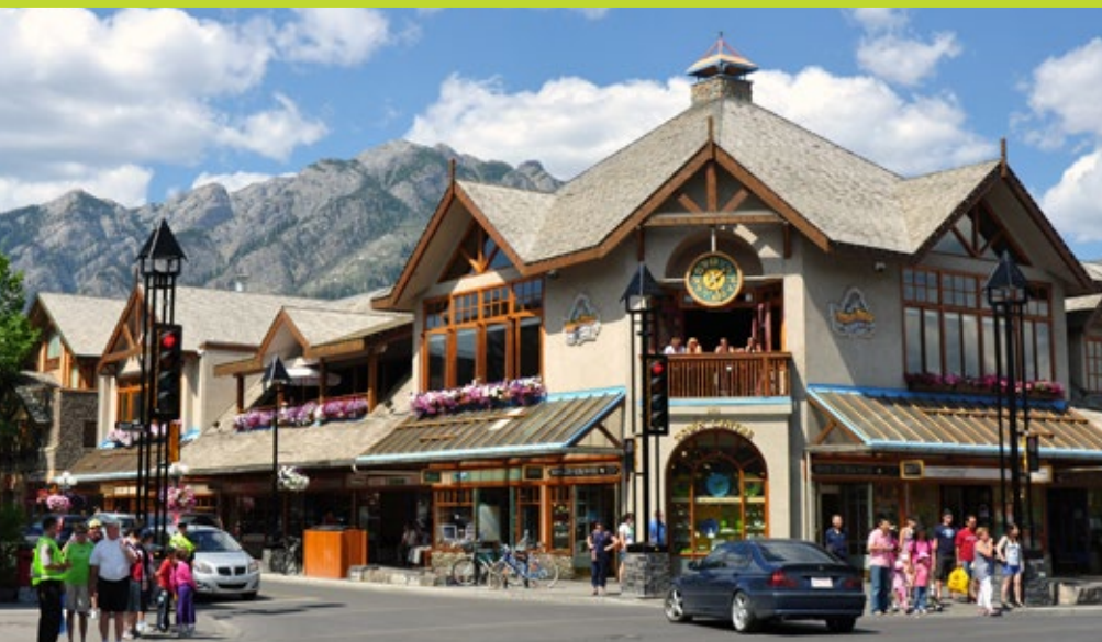
Figure 19: Example of building with active facades on the street and avenue
