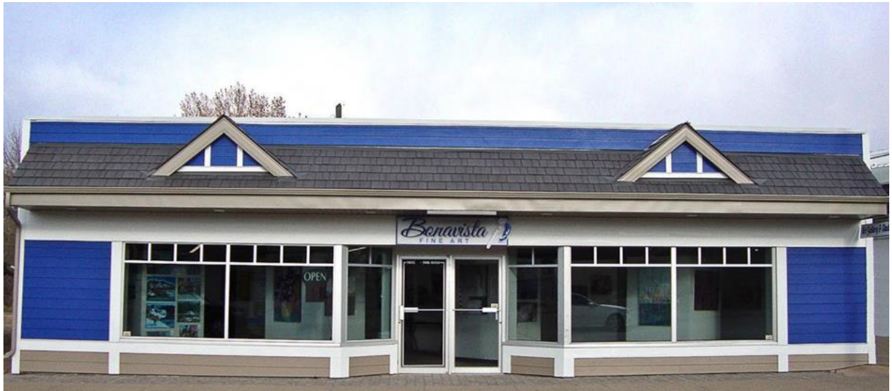
Figure 8: Bonavista Fine Art is a good example of enhanced storefronts through placemaking.
