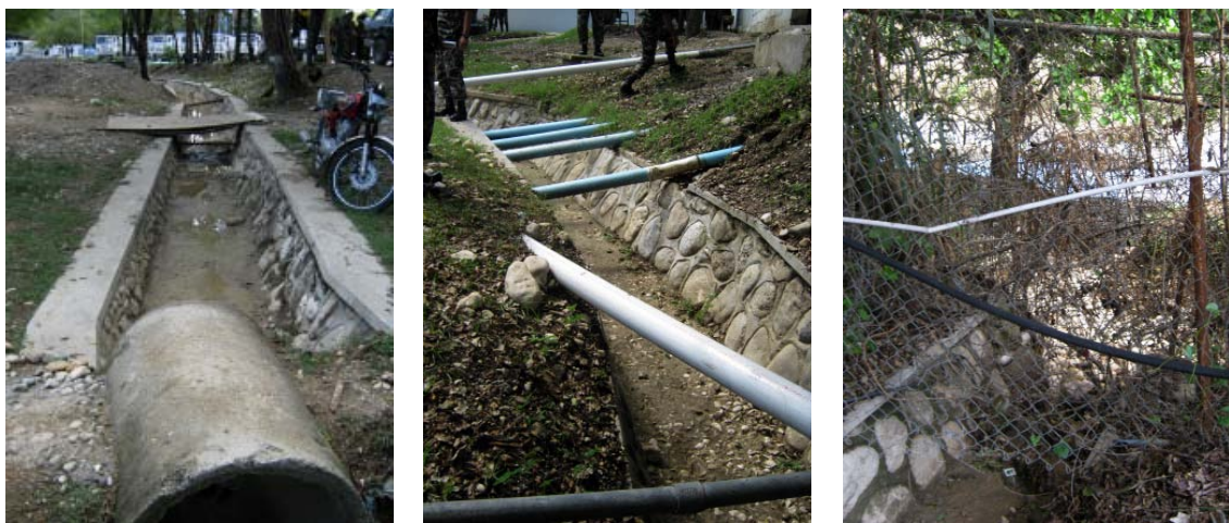
Figure 10: Canal through Camp, Pipes over Canal, Canal Flowing into Meye Tributary
