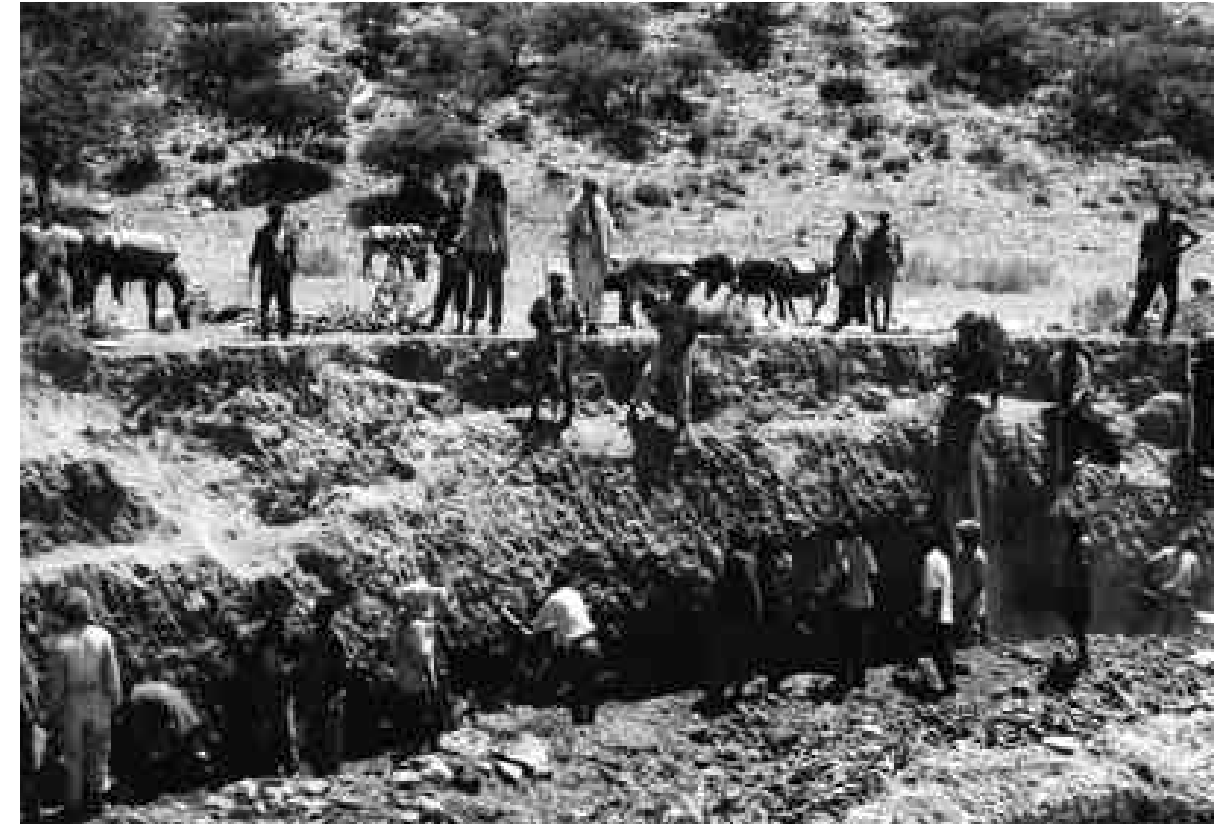
One of the many self-help groups in Tigray, Ethiopia, visited by Nick Chisholm in September last. These villagers construct an irrigation channel
