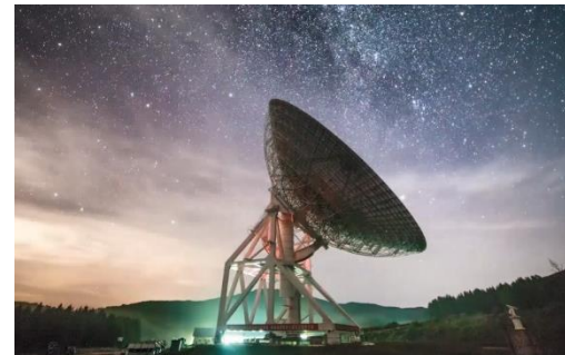
Ground Support and Application Facilities
