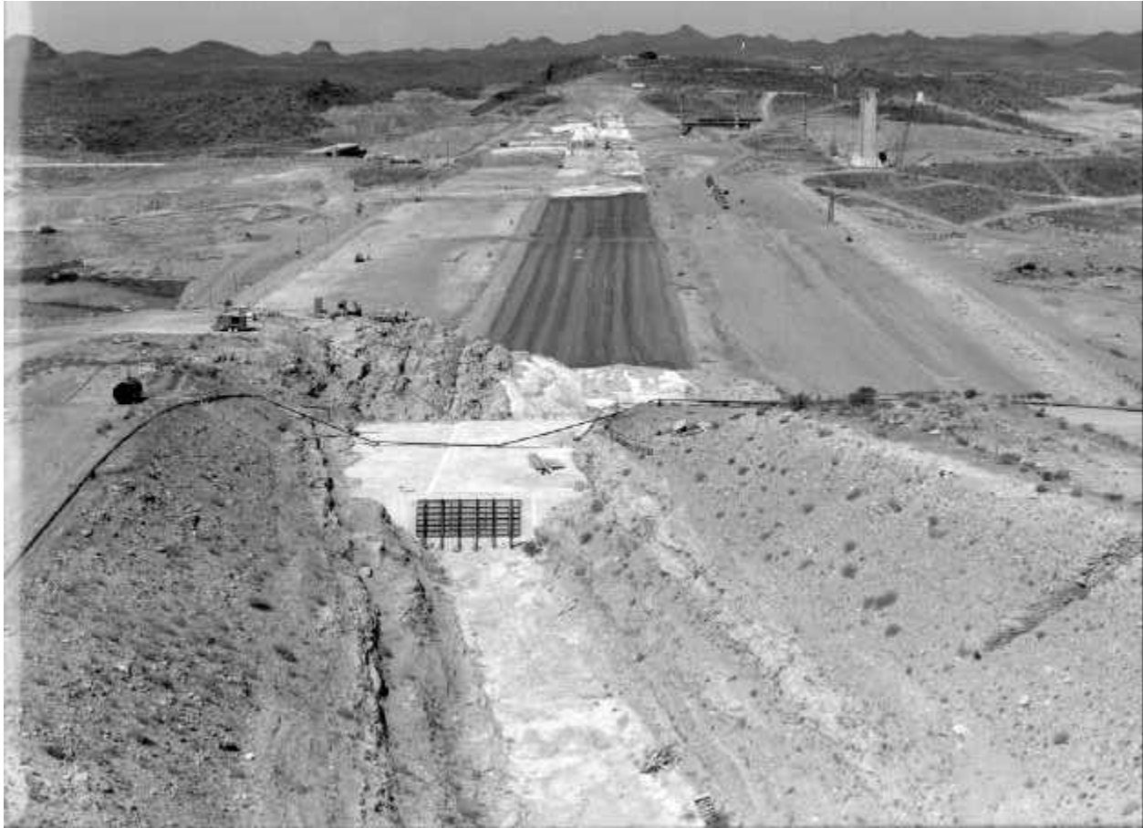
Figure 23 - New Waddell Dam Construction
