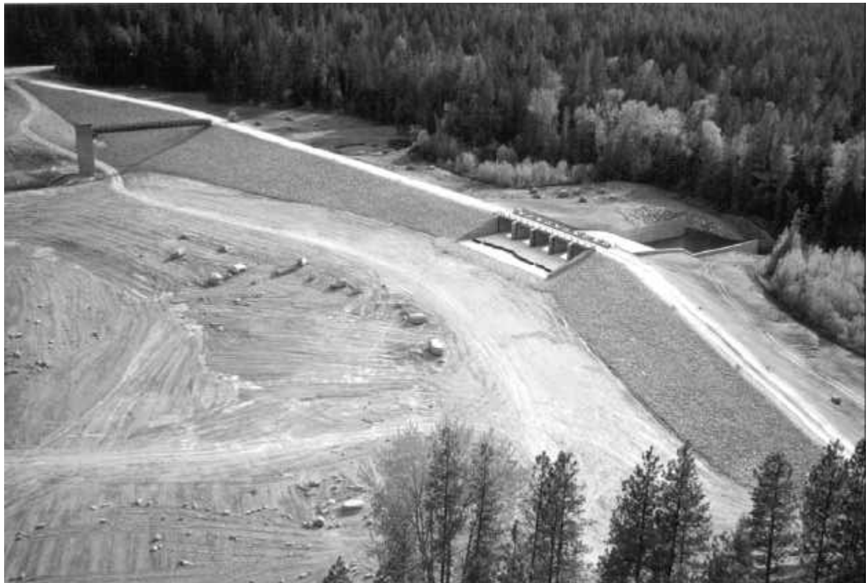
Figure 22 - McDonald Dam - New Dam in 2000
