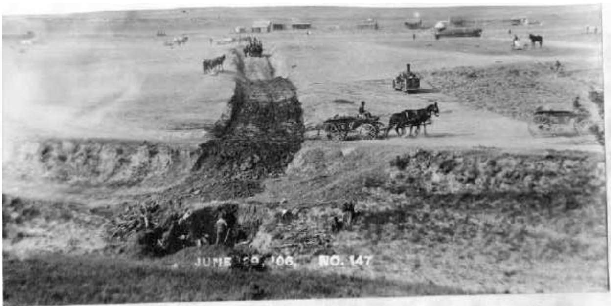
Figure 6 - Belle Fourche Dam - Cutoff Trench Construction
