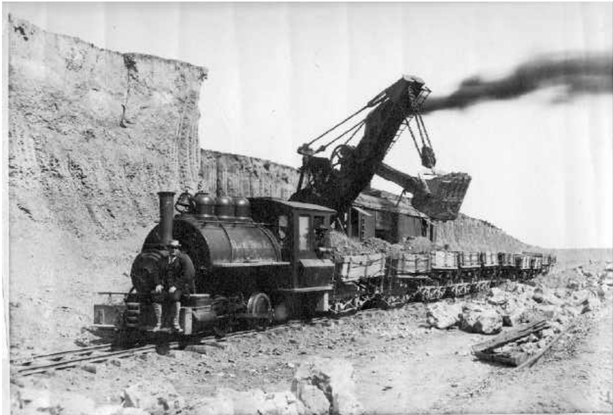
Figure 7 - Belle Fourche Dam Steam Shovel, Dinkey Locomotive, and Train of Side-Dump Cars in Borrow Pit
