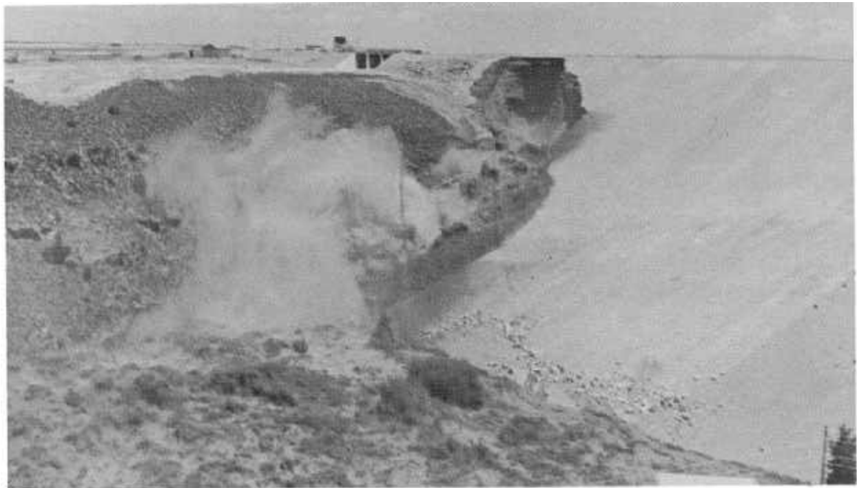
Figure 27.—Dam crest breaching 11:55 a.m., June 5, 1976.
