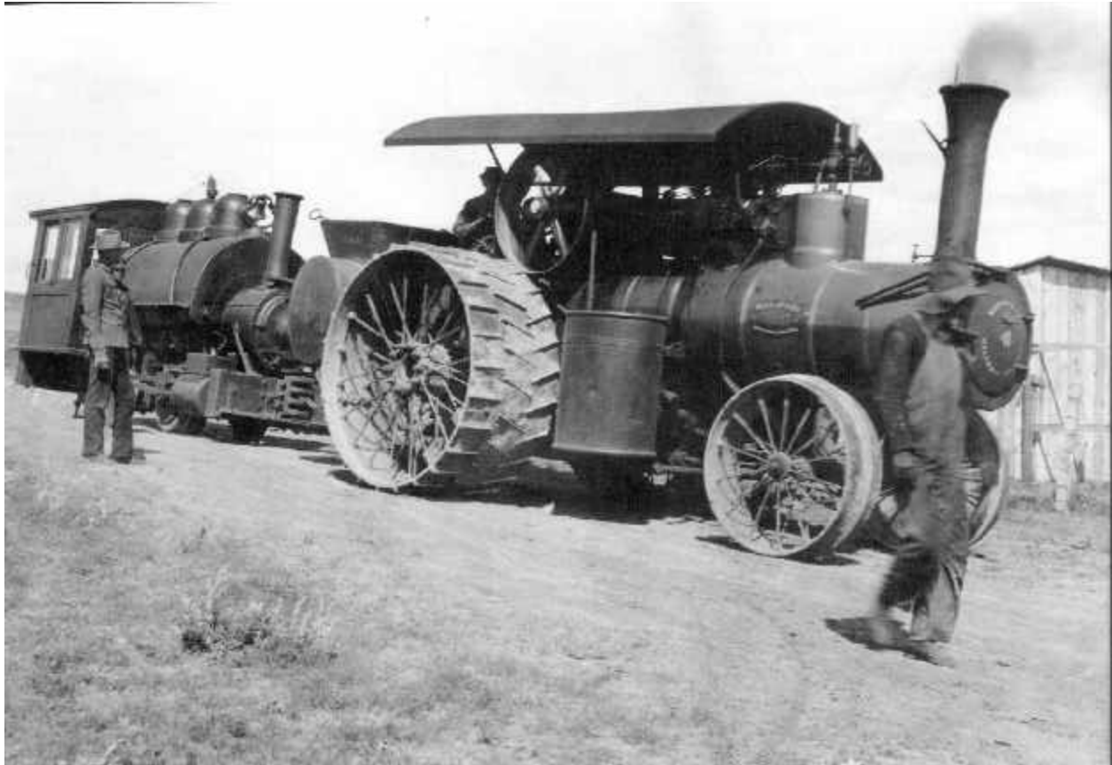
Figure 9 - Belle Fourche Dam - Traction Engine Hauling Dinkey Locomotive to Damsite
