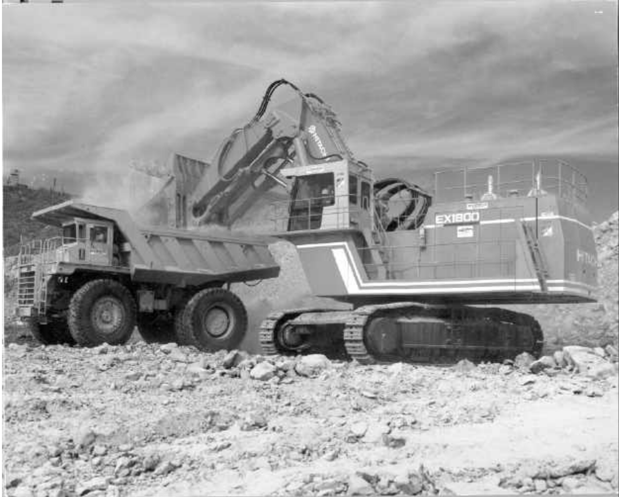
Figure 24 - New Waddell Dam - Construction Equipment
