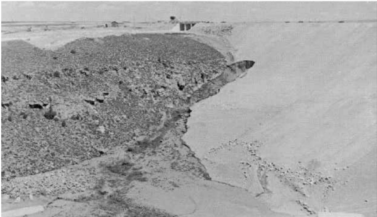
Figure 23.—Dozers lost in leak at El. 5200.
