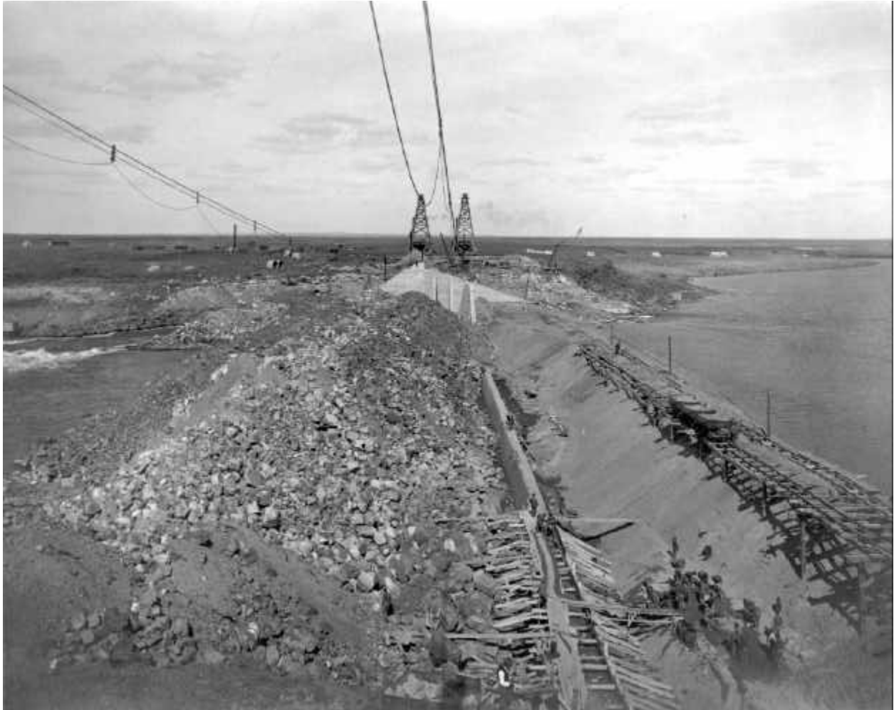
Figure 4 - Minidoka Dam Construction
