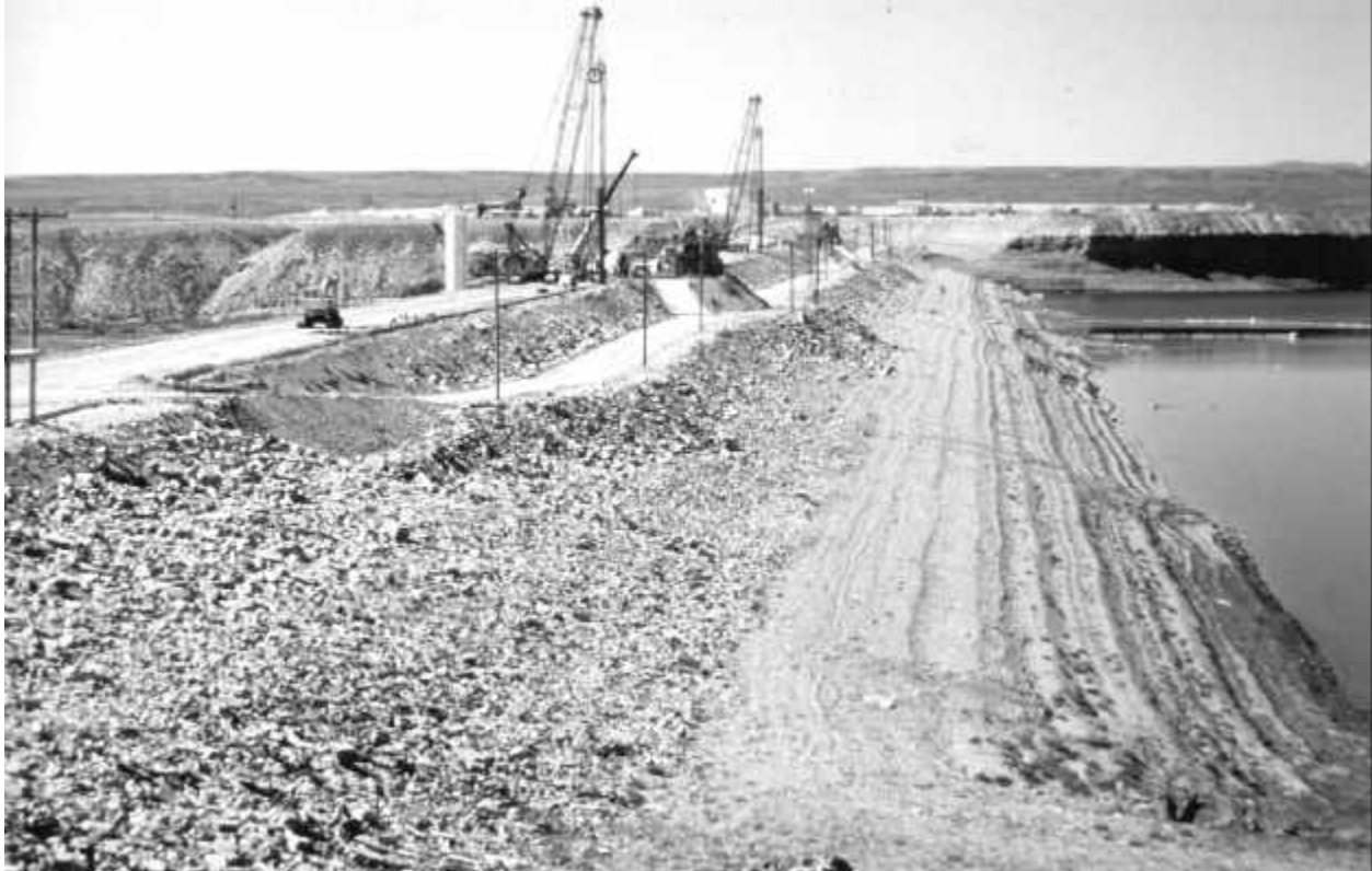
Figure 19 - Fontenelle Dam - Diaphragm Wall Construction
