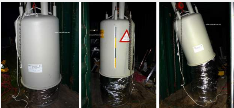
Figure 2. The 'Vacuum Chamber' is raised and removed.
