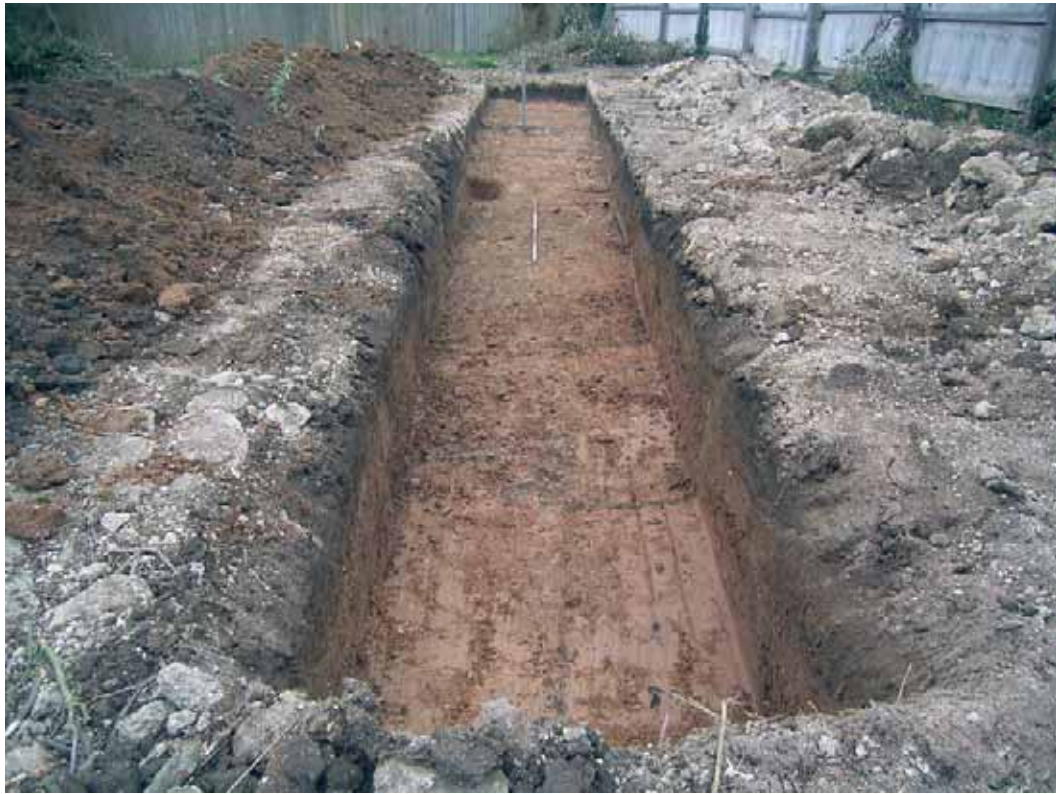
Plate 1: Trench 1 from the south east
