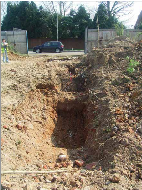
Plate 5: Trench 4 from the north-west
