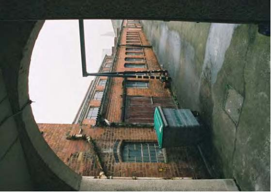
Plate 13: Internal yard of former Blakenhall Japan works
