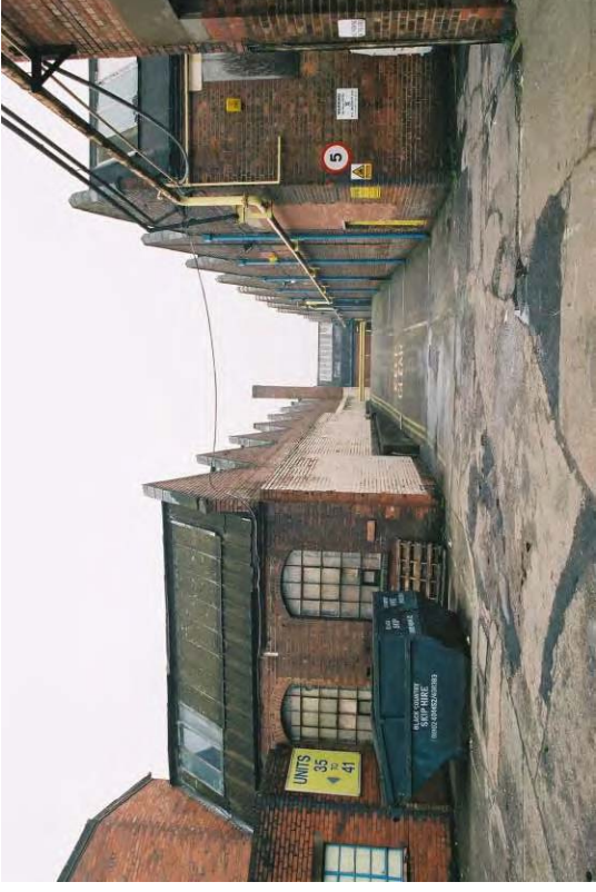
Plate 17: Access road between major workshop ranges
