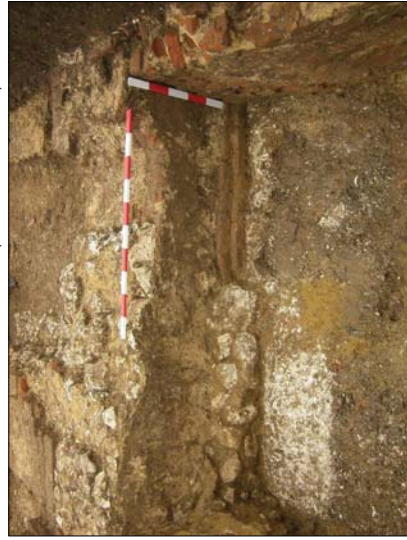
Plate 6: North facing elevation showing blocking wall 210 within the archway in wall 208 of cellar of Great Hall (scales 1m and 0.5m)
