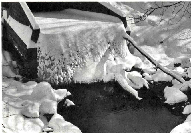
Culvert holds it back . . .
