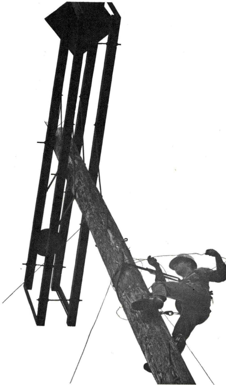
A1C. Dennis A. Cierpial, 905th Communications Flight, puts the finishing touches on the installation of an inverted "V" antenna 50 feet above the 439th avionics building. The operation is part of his duties as an outside plant telephone installer during the May UTA. The antenna is a cog in the 905's ground radio communications network.
