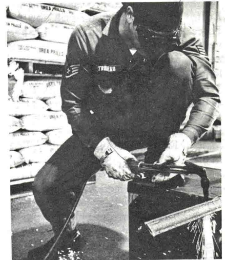
SSgt. Robert Trudeau, 905 CEF, uses a blow torch to cut a piece of angle iron which will later be drilled and used to reinforce two revetments.
