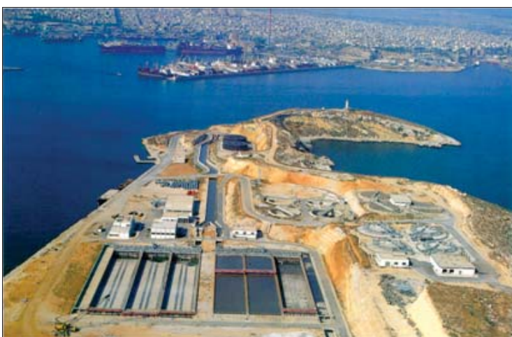
Fig. 7. Wastewater treatment plants protect both human health and the vulnerable marine environment (© United Nations Environment Programme/Mediterranean Action Plan)
