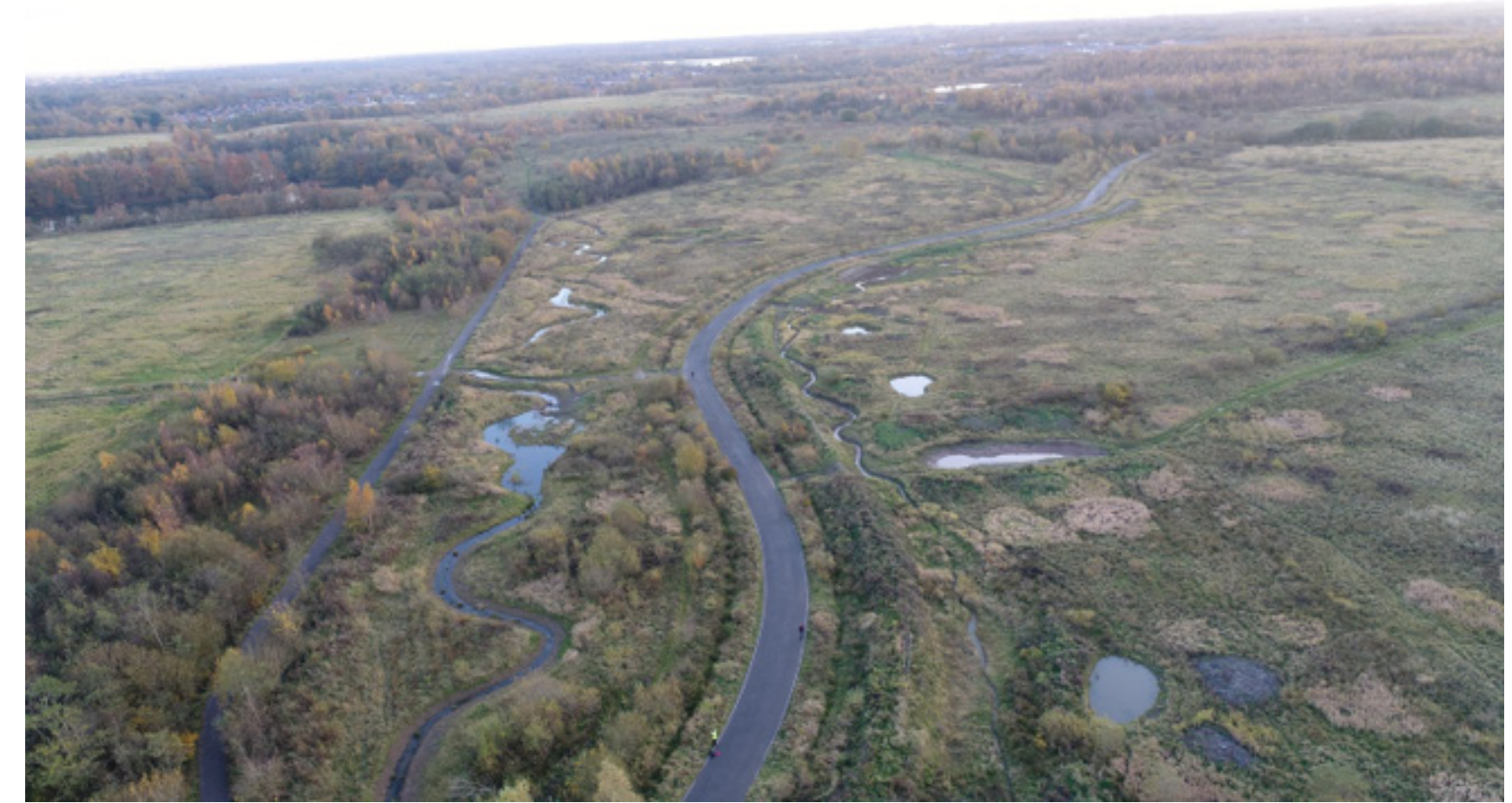
Aerial view of the Bickershaw 'slow the flow' site Image © Tony Da Silva, Wildlife Trust for Lancashire, Manchester and North Merseyside
