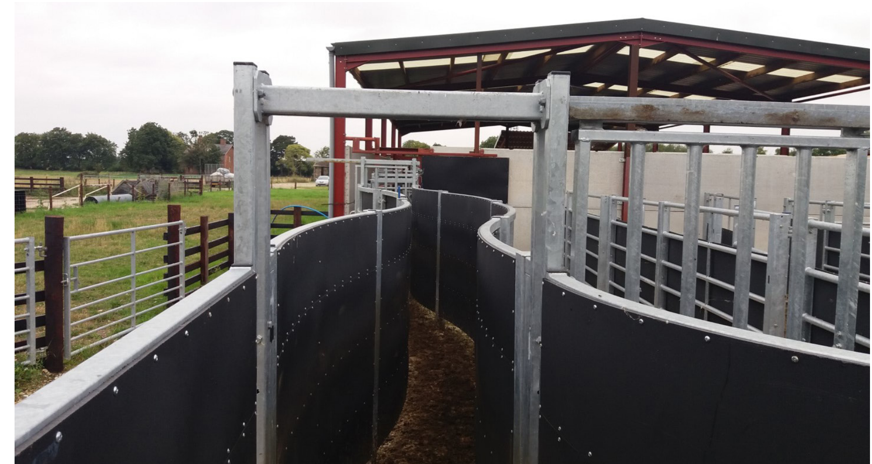
New livestock welfare facilities at Woodhall Spa Airfield Nature Reserve Image © Lincolnshire Wildlife Trust
