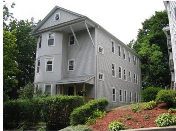
Converted small apartments: A three-decker in Worcester that has been converted into three condos. Three-deckers are distinct for not only their age, but their similar rectangular shapes and clapboard sidings. Credit: Redfin.
